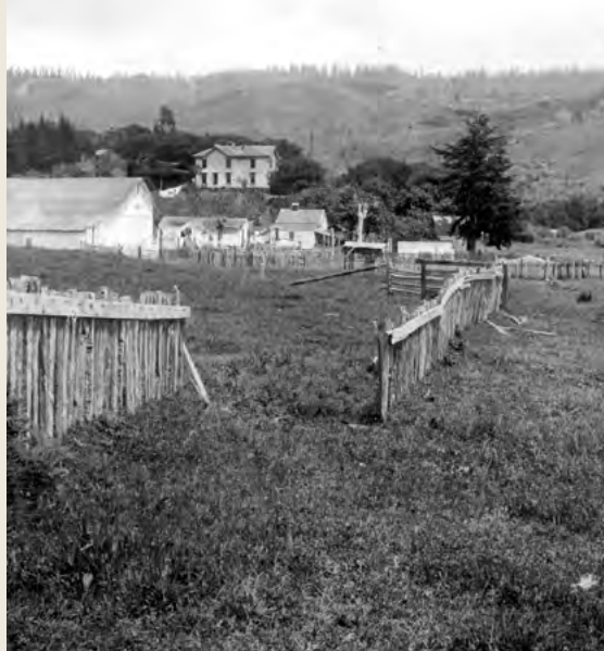
Effects of the 1906 San Francisco earthquake
