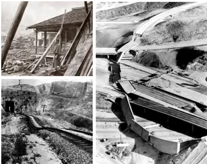
Damage caused by earthquakes
