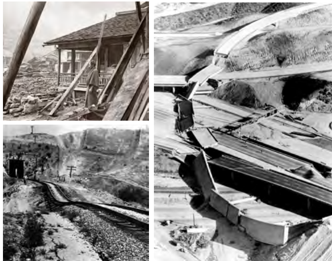
Damage caused by earthquakes
