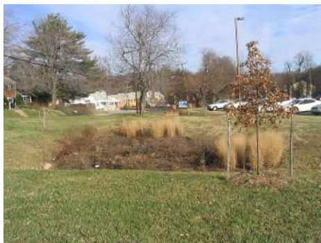
Figure 8.10: Intercepting nonpoint pollution between the source and waterway has been found to be successful. Pictured here, a bioretention cell, or rain garden, in the U.S, is designed to treat polluted storm water runoff from an adjacent parking lot.
