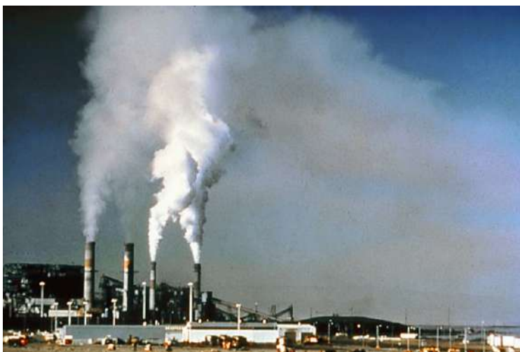
Figure 8.2: A major source of air pollution is the burning of fossil fuels from factories, power plants, and motor vehicles. Photo was taken prior to installation of emission controls equipment for removal of sulfur dioxide and particulate matter.
