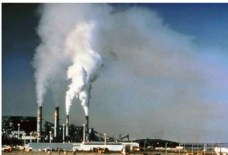
Figure 5.4: A power plant and its emissions before emission control equipment was added.
