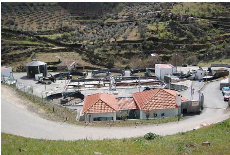
Figure 3.21: Wastewater Treatment: Most wastewater treatment facilities separate contaminants from water by passing wastewater through a series of settlement containers. At each step, solids and particles are separated from water. Chemical and biological agents are also used to remove any remaining impurities.
