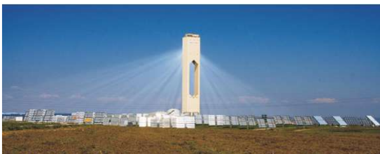
Figure 1.8: This solar power plant uses mirrors to focus sunlight on the tower in the center. The sunlight heats a liquid inside the tower to a very high temperature, producing energy to make electricity.
