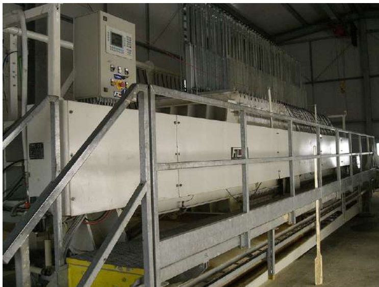
Figure 8.12: Sand processing Mill, near Provodin, Czech Republic. Water is used to wash mined sand, then is drained into tanks, filtered, and recycled.
