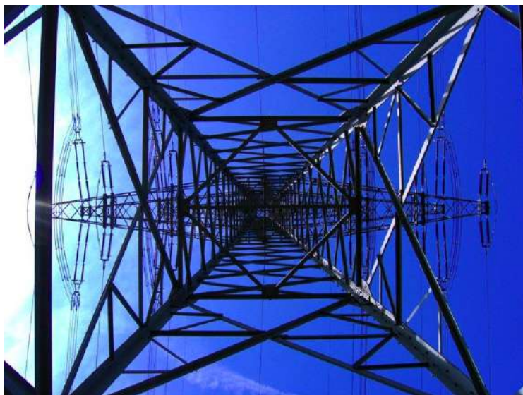
Figure 1.1: Electrical transmission towers like the one shown in this picture help deliver the electricity that you use for energy every day.
