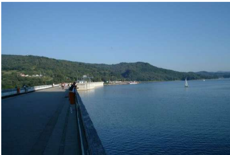
Figure 3.5: Industrial water use: A power plant in Poland sits on the edge of a lake with easy access to water for cooling and other purposes.
