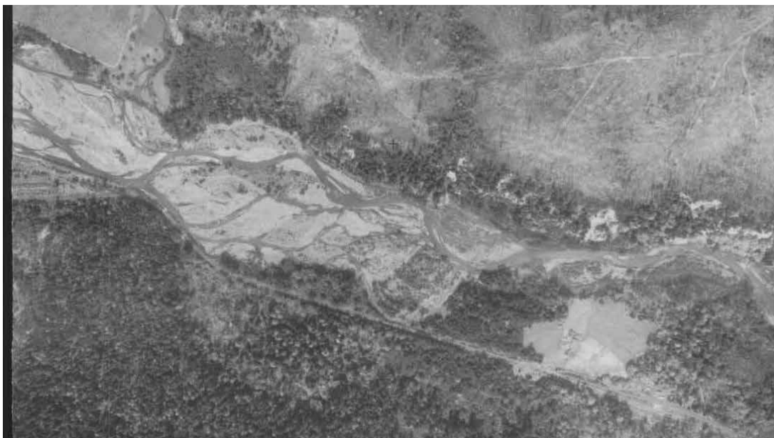
Figure 8: Alward Road Reach on the Carbon River, 1931 Source: Pierce County
