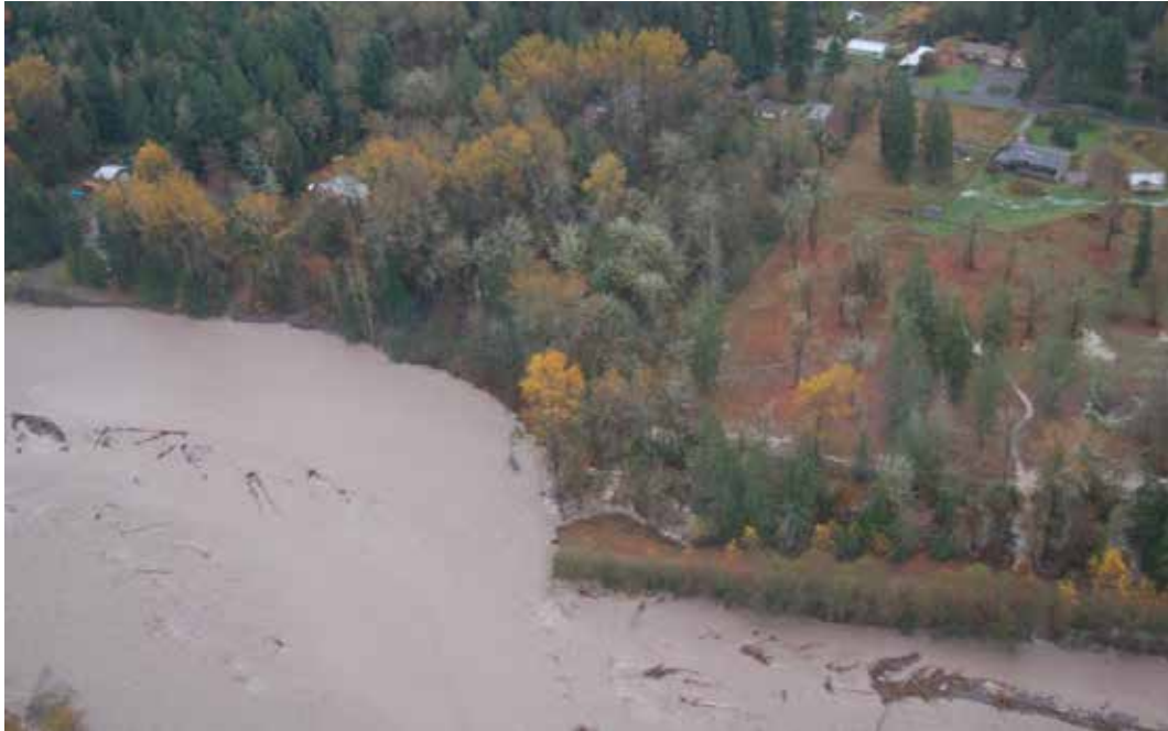
Figure 9: Levee Breach at Alward Road, 2006 Source: Pierce County
