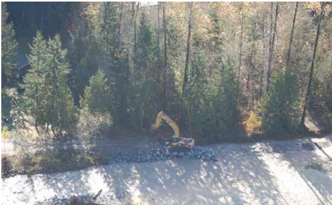
Figure 10: Repairing a Levee at Alward Road Source: Pierce County
