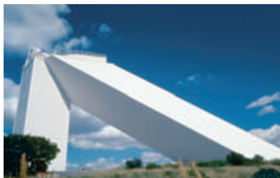
Figure 11 The McMath-Pierce Solar Telescope at Kitt Peak Near Tucson, Arizona. Movable mirrors at the top follow the sun, reflecting its light down the sloping tunnel.
