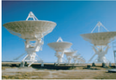
Figure 8 A The 43-meter Radio Telescope at Green Bank, West Virginia The dish acts like the mirror of a reflecting telescope, focusing radio waves onto the antenna. B The Very Large Array Near Socorro, New Mexico Twenty-seven identical antennas operate together to form this radio network.
