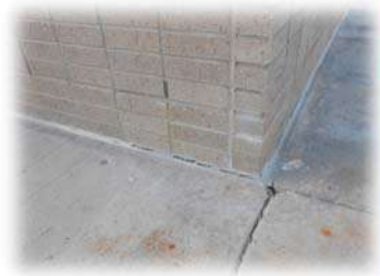
Cracking concrete
