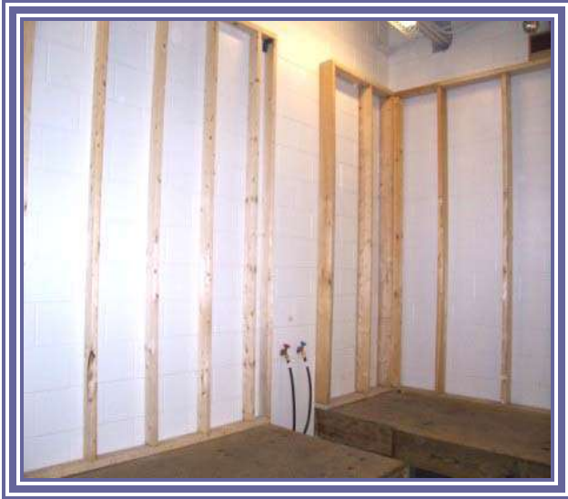
Plumbing classroom being prepped to begin labs
