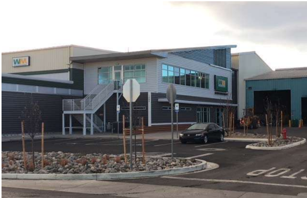
Sage Transfer Station, near downtown Reno
