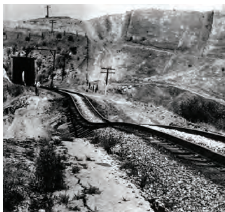
Damage caused by earthquakes
