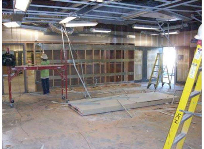
2. Installation of casework backing and drywall on-going.
