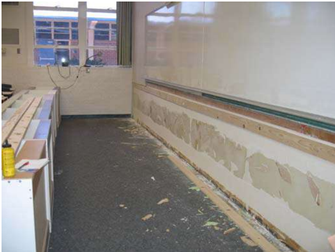
3. Building B- Casework backing complete, ready for installation.
