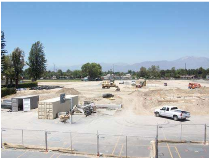
3. Site overview- Work in progress.
