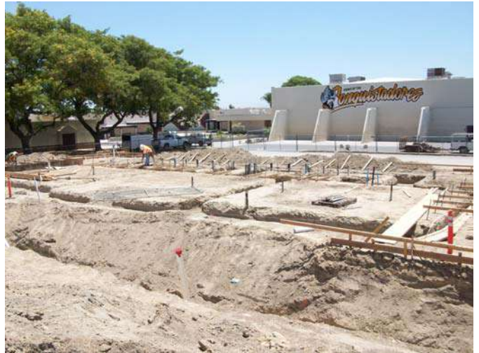
2. Building B- Setting form work has begun.
