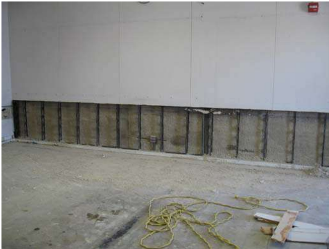
1. Building A- Open wall ready to receive casework backing.
