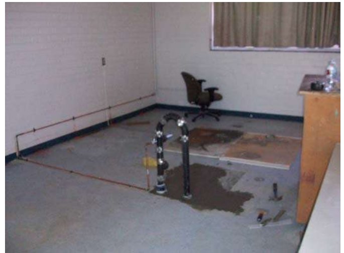
2. Building B- Rough-in plumbing in classroom 16 complete.
