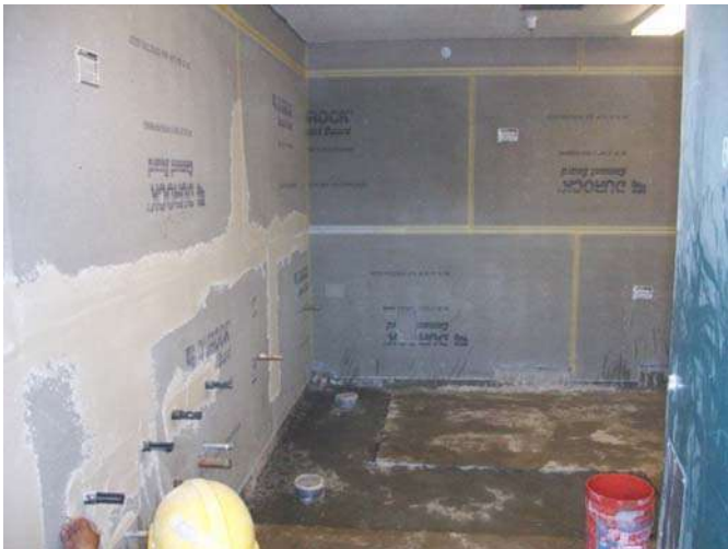
3. New backer board at restroom complete.
