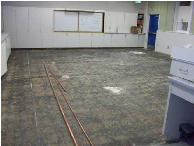
3. Home Economics Bldg.: Removal of existing flooring complete.
