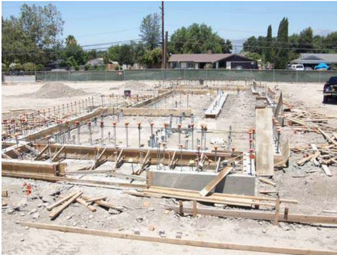
1. Building A- Removing form work.
