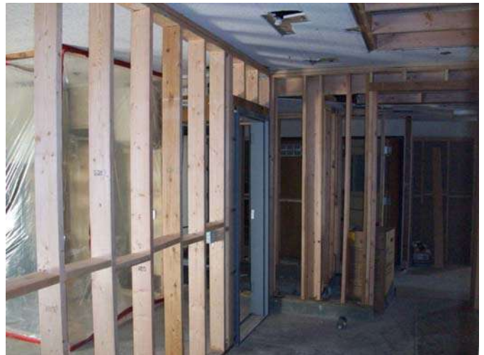
4. New wood walls and HM frame complete.
