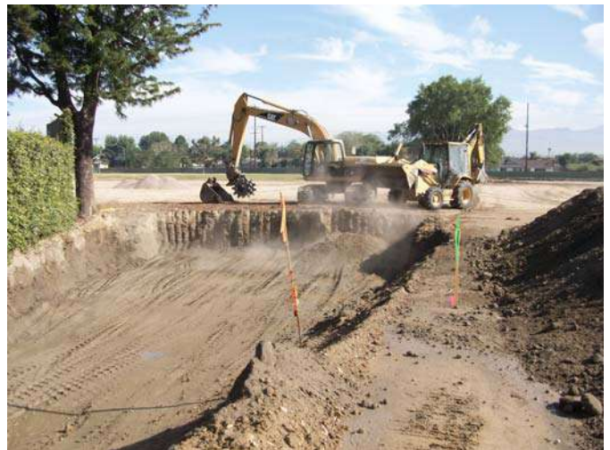
4. Over-excavation for stair bleachers. .
