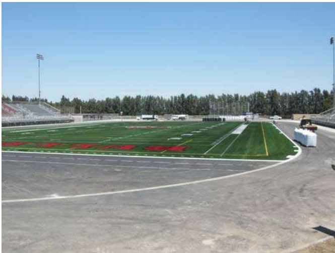
1. Ayala HS- New field turf has been installed.
