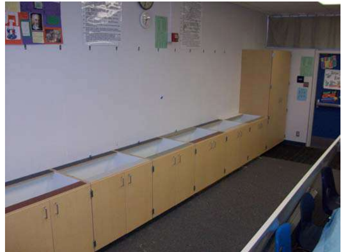
4. Building B- Installation of classroom casework has begun.
