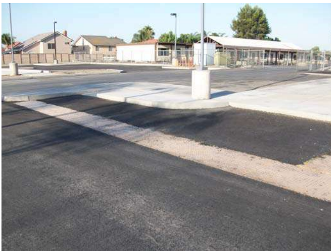
3. New asphalt paving looking south.
