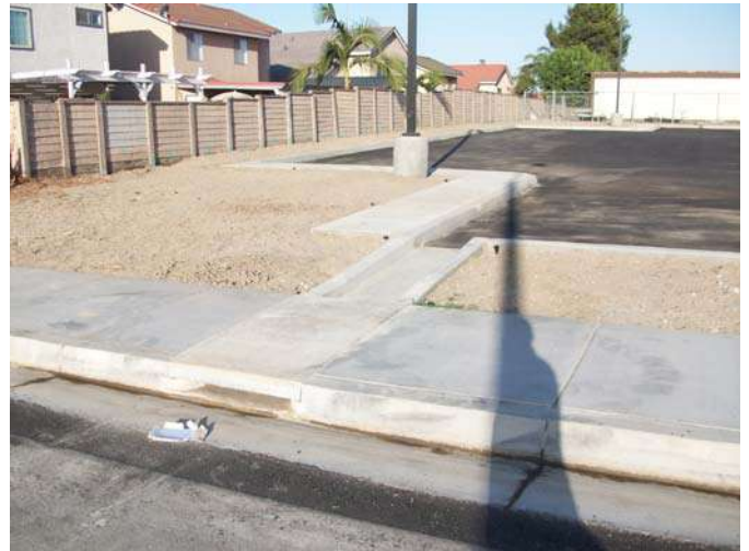
2. New concrete culvert and irrigation system installed.
