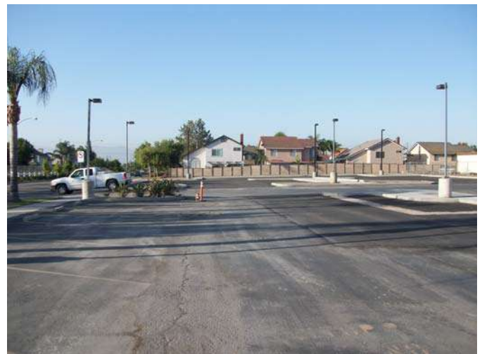
4. New light poles have been installed.
