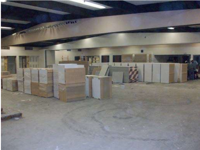
1. New casework cabinets have been delivered.
