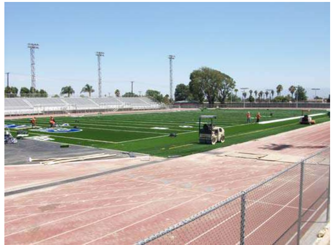
2. Chino HS- Installing new field turf material
