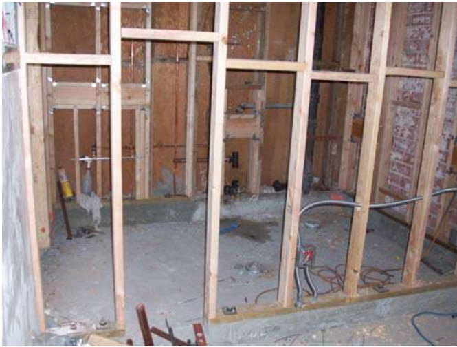
1. Home Economics Bldg.- Rough-in electrical and plumbing complete.
