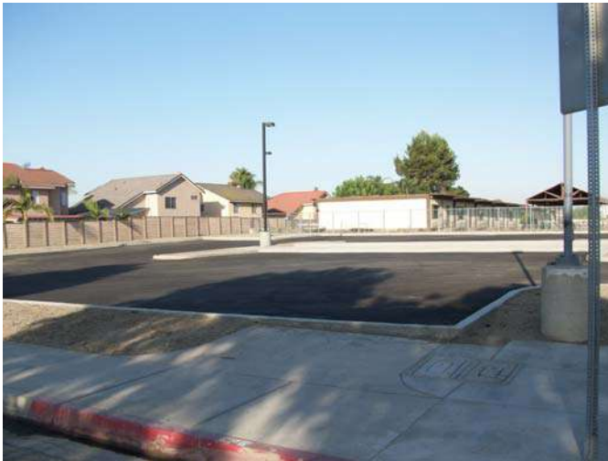
1. New asphalt paving looking west.
