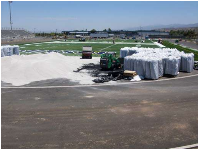
3. Chino Hills HS- Applying sand on the new field turf.
