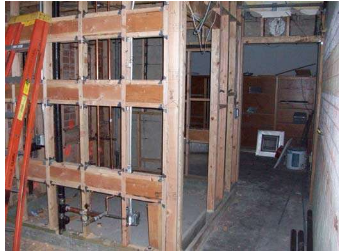
2. Counseling Bldg.- Rough-in electrical and plumbing complete.
