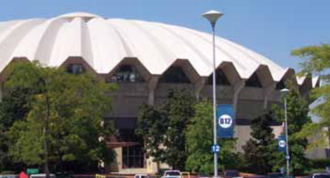
West Virginia University Coliseum features an ELASTOSPRAY® roofing system.
