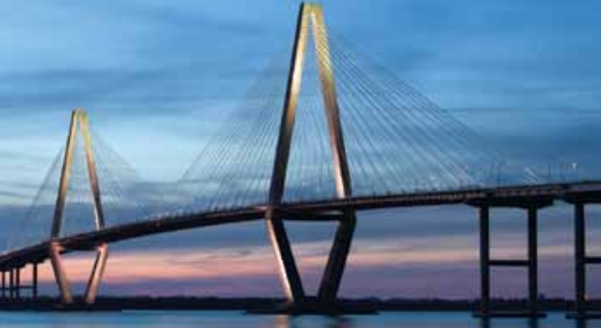
Cooper River Bridge features a BASF latex-modified concrete bridge deck overlay.
