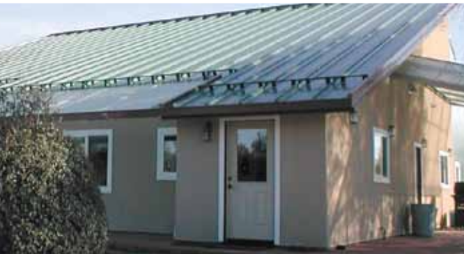
The Habben Home is built with structural insulated panels made with BASF polyurethane insulation.
