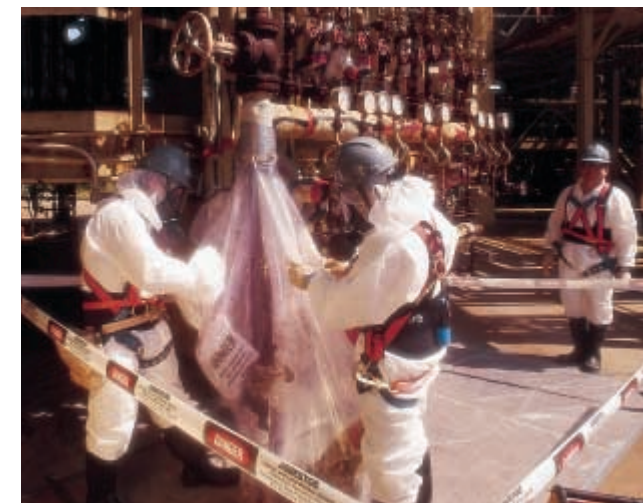
Figure 11.12 Asbestos was formerly used to insulate buildings. It is now known to cause lung cancer and other lung diseases and must be removed from these buildings, as shown here.
