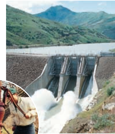
A dam and a pump regulate the flow of water.
