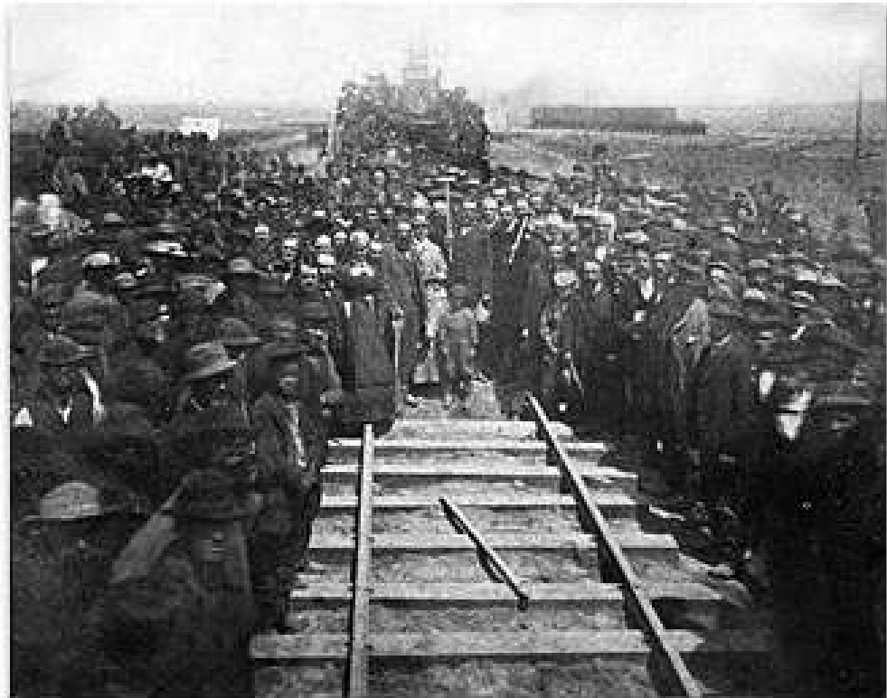
The Last Rail is Laid
