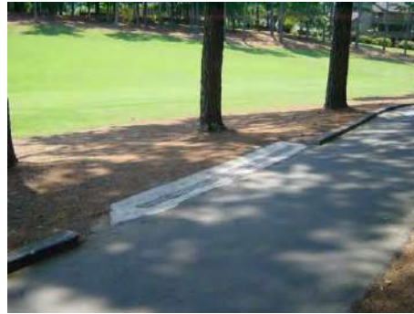
(Right) - Adding drainage via catch basin or slot drain in low spots is often required .
