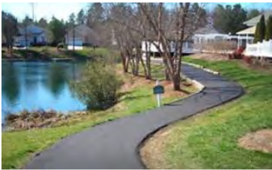
Left - Retrofitting cart paths involve restoring shoulders for drainage.
