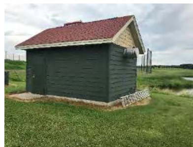
Pump house and station controls
