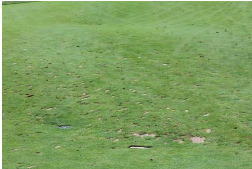
Above -The unintended fairway collection area on the 14th hole. The catch basin is undersized for the drainage area, and typical of the drainage system
