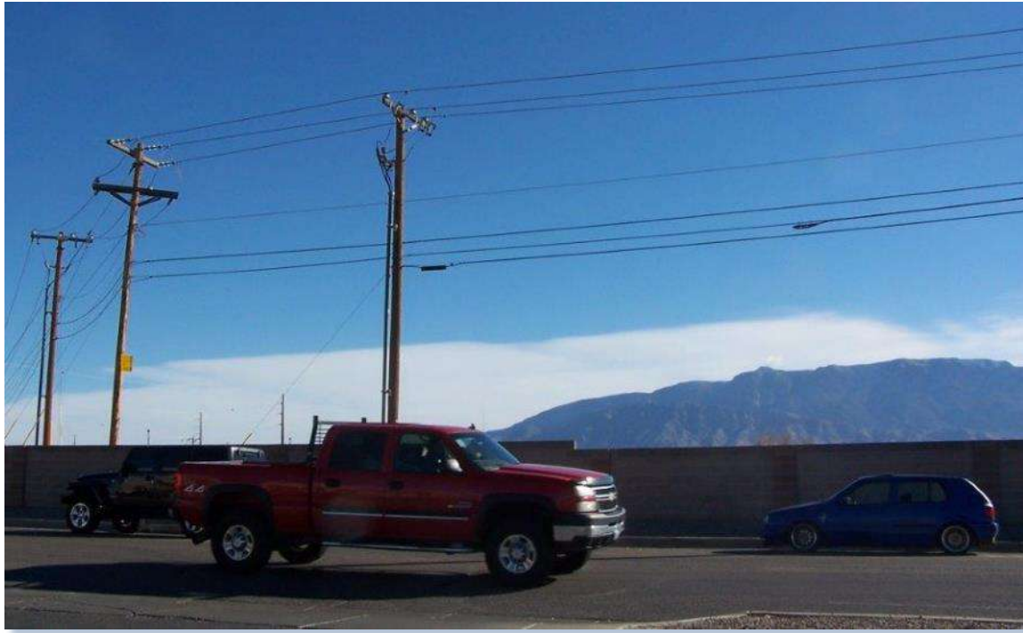
Figure 46: Rio Rancho Copper Telephone Lines
