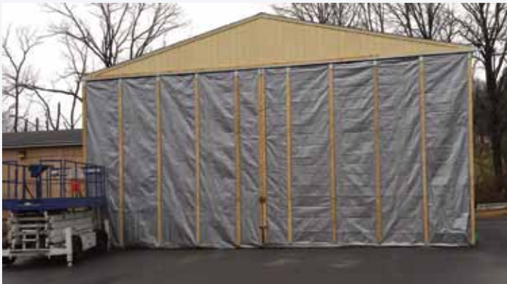
This salt shed entrance curtain keeps rain from getting inside a salt shed and contaminating stormwater runoff. Whitehall Township, Lehigh County, 2017 First Place Winner
