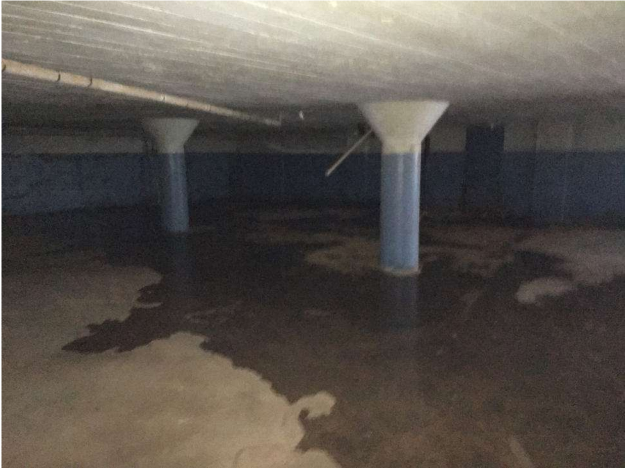
Lower Level – southern section
