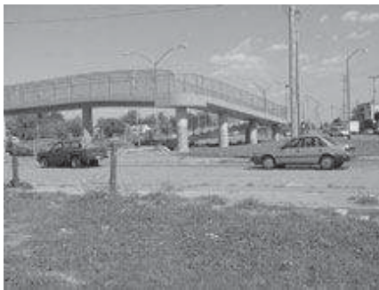
Pedestrian bridge, south of I-90
