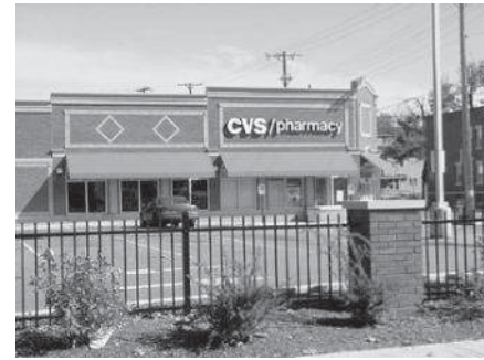
CVS at Madison Avenue and West Boulevard
