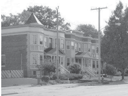
Rowhouses on West 117th Street.
