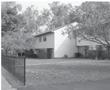
Area 2: Housing near Recreation Center
