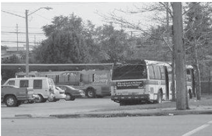
Existing RTA station from Madison Avenue
