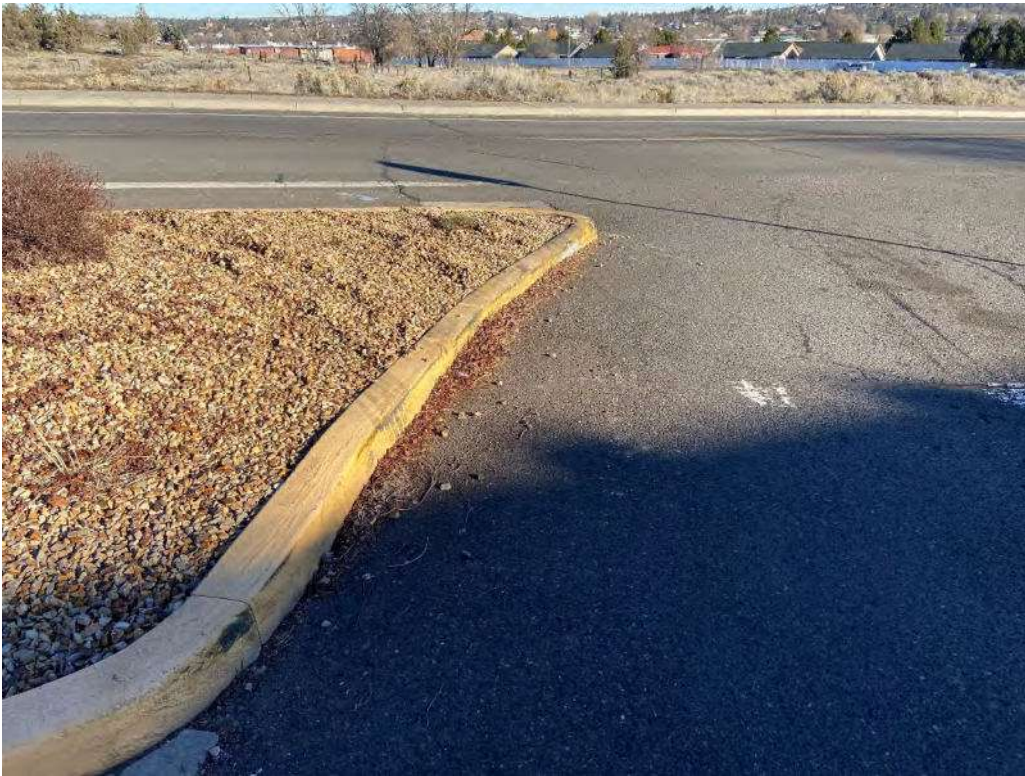
Figure 5. Curb condition of separator at stop bar at J Street/Strawberry Lane intersection
