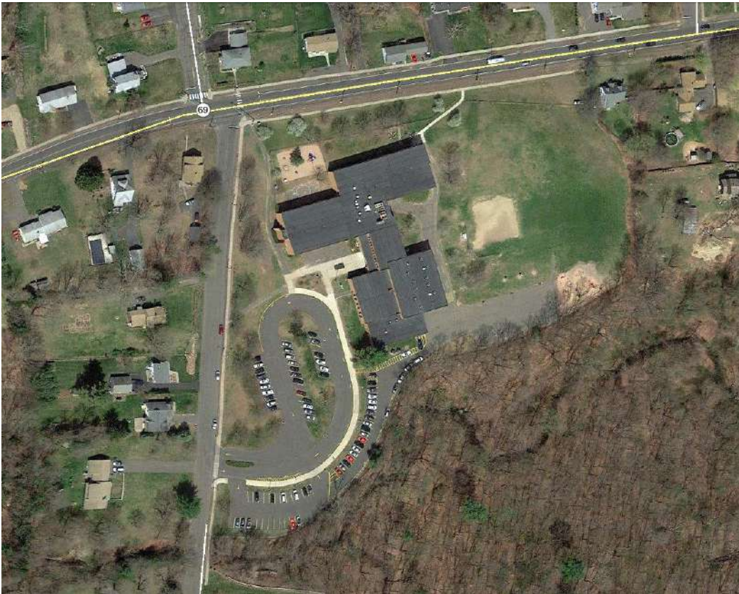
South Side Elementary School, aerial photo of site
