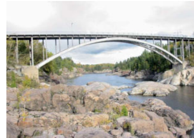
Arvida Bridge, Canada
