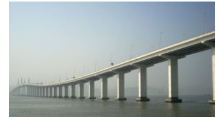
Hong Kong-Zhuhai-Macau Bridge, Hong Kong
