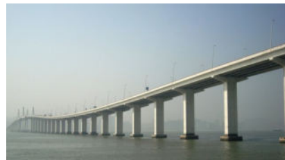
Hong Kong-Zhuhai-Macau Bridge, Hong Kong
