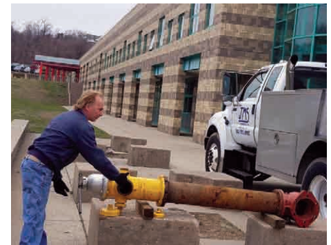
What does it take to remove a fire hydrant?
