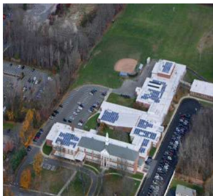
Newtown Middle School solar project completed in 5/1/13 Size of System: 180,000 Watts
