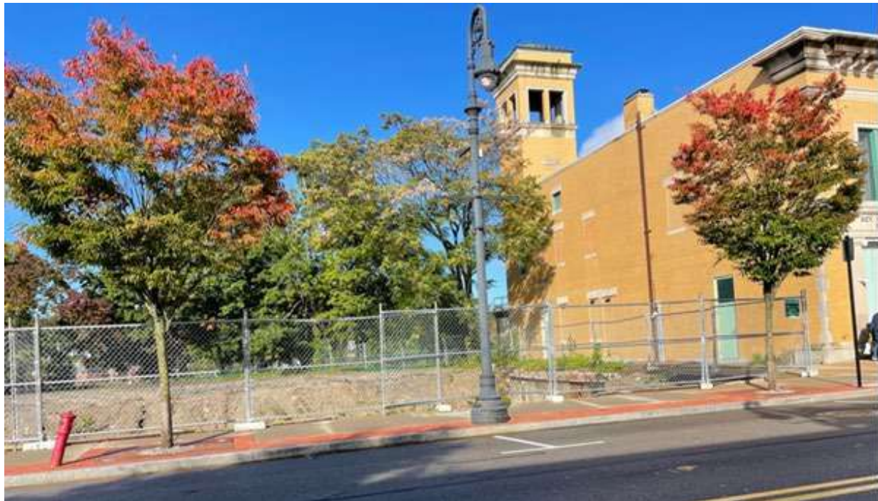
View of the northern portion of the Project Site
