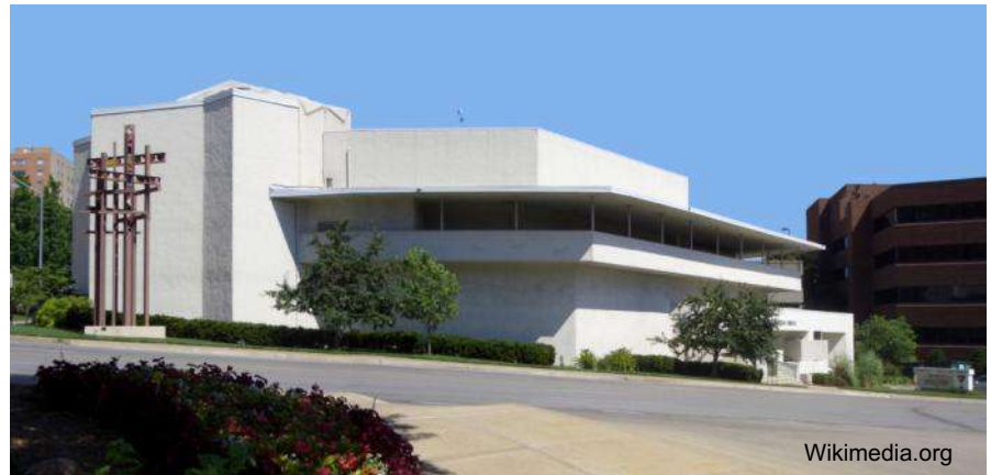
Community Christian Church Kansas City, MO Architect: Frank Lloyd Wright, 1940
