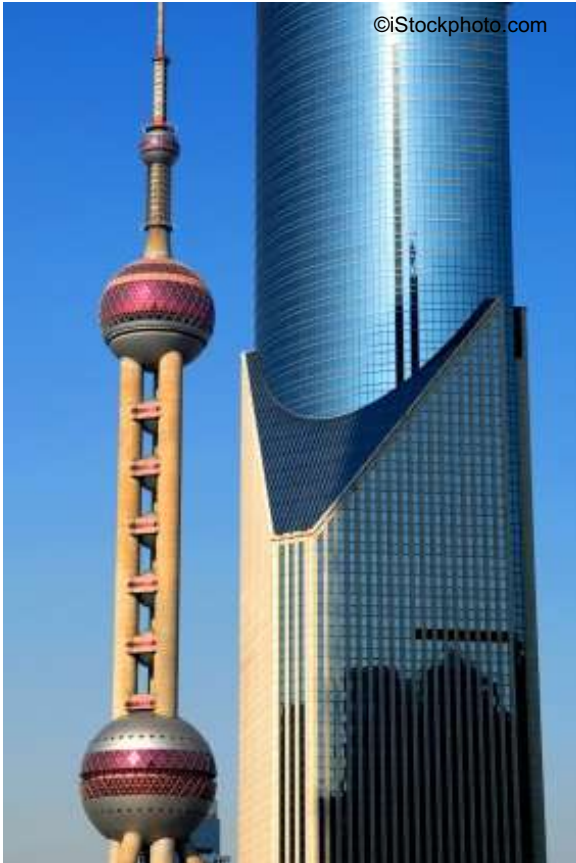
Oriental Pearl Tower Shanghai Architect: Jiang Huan Cheng, Shanghai Modern Architectural Design, Co.
