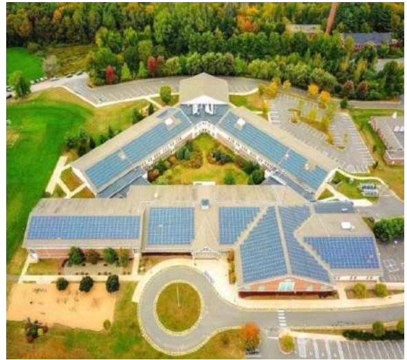
Reed Intermediate solar project completed 8/1/17 Size of system: 635,000 Watts
