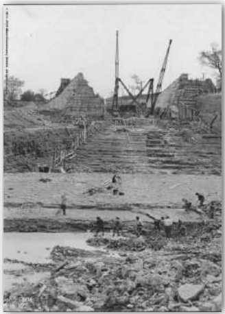
Constructing Huffman Dam Miami Conservancy District Photo Collection
