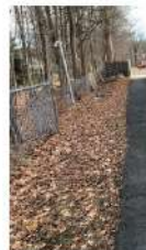
D.2.2: Walkways / Site Stairs
