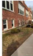
D.2.1: Walkways / Site Stairs
